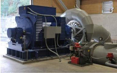
The James Leffel & Co has used Alab for hydraulic design of a new hydro turbine replacing an outdated turbine in the Redwood River in the American state of Minnesota and has significantly enhanced the power generating ability.
